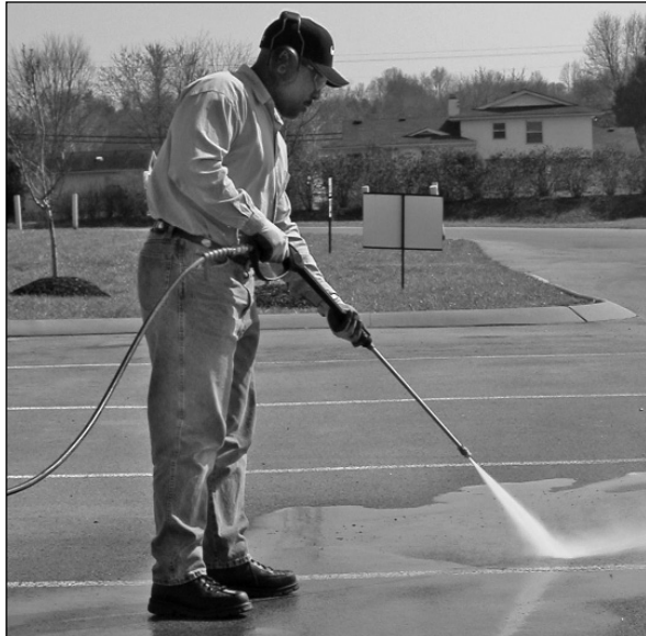
Figure 14 - Optimum angle to cleaning surface
